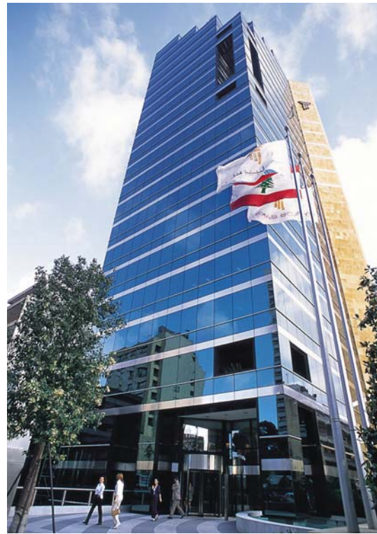
Banque Byblos, Liban
